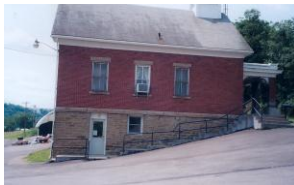
Whiteley Township Municipal Building
