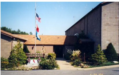
Jefferson VFD Building
