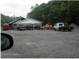
Springhill Township Municipal Building
