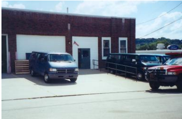
Central Greene School Warehouse
