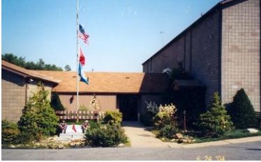
Jefferson VFD Building
